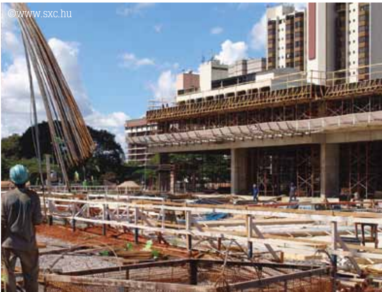
Urban construction site
