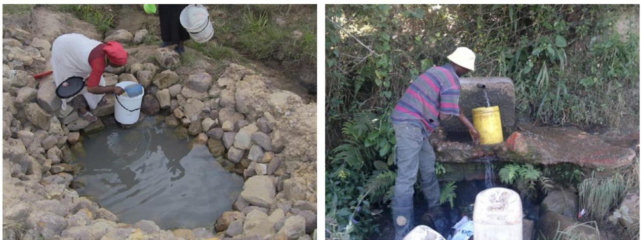
Figure J.8: An open spring (L) and a protected spring (R)
