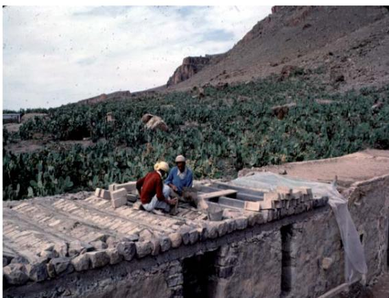
Figure 4: Construction of flat roof by self-builder with instructor
