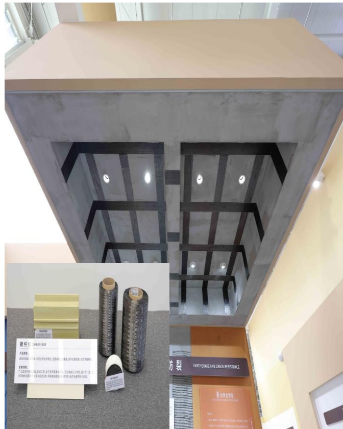
Carbon fiber materials can increase structural load-bearing capacity by 30%-50%.
