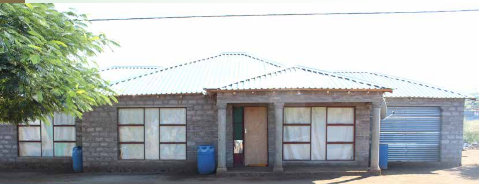
The house of Wilson Mokoena from Ga- Malokela Village (Burgersfort), Tubatse Local Municipality, Limpopo who used the rural loan fund to build a new house
