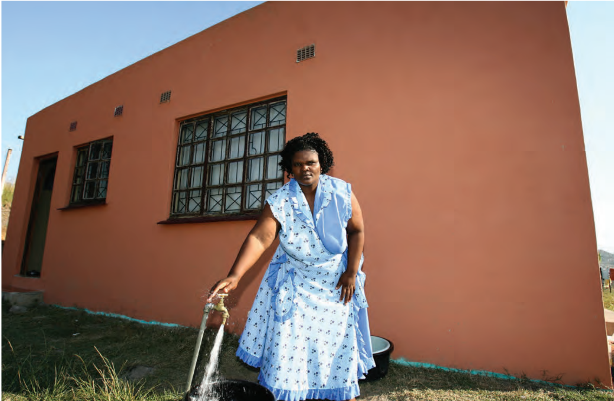
Zanele Mthethwa is one the satisfied beneficiaries of home loan funding made possible by the RHLF. Here she is seen standing in front of her refurbished house at KwaHlomendlini, Mandeni, in KwaZulu-Natal.
