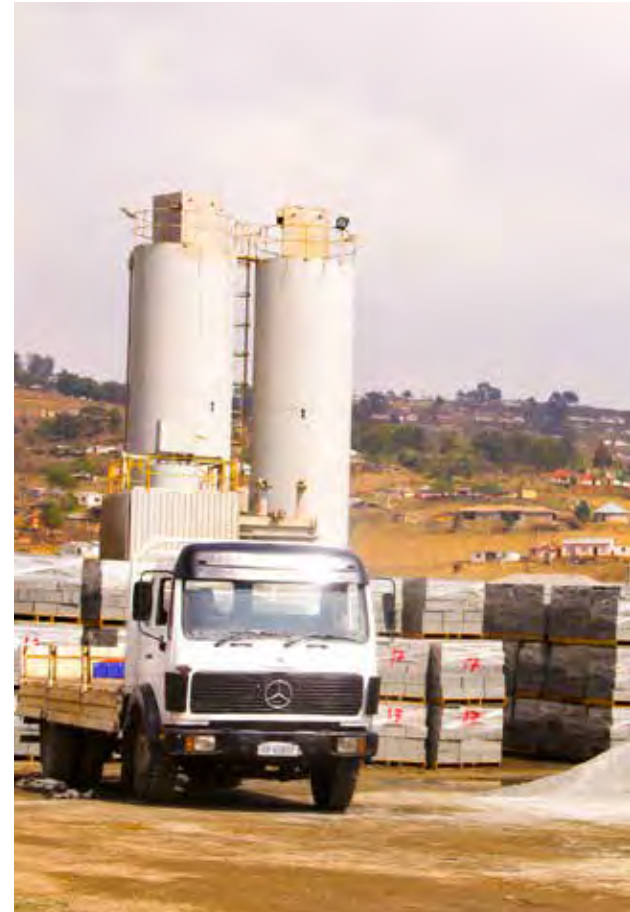
Construction site at Vulindlela rural project
