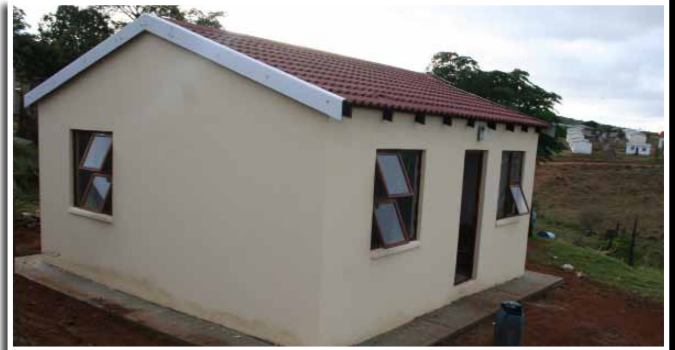
A house built in Moses Mabida, Kirkwood, Eastern Cape
