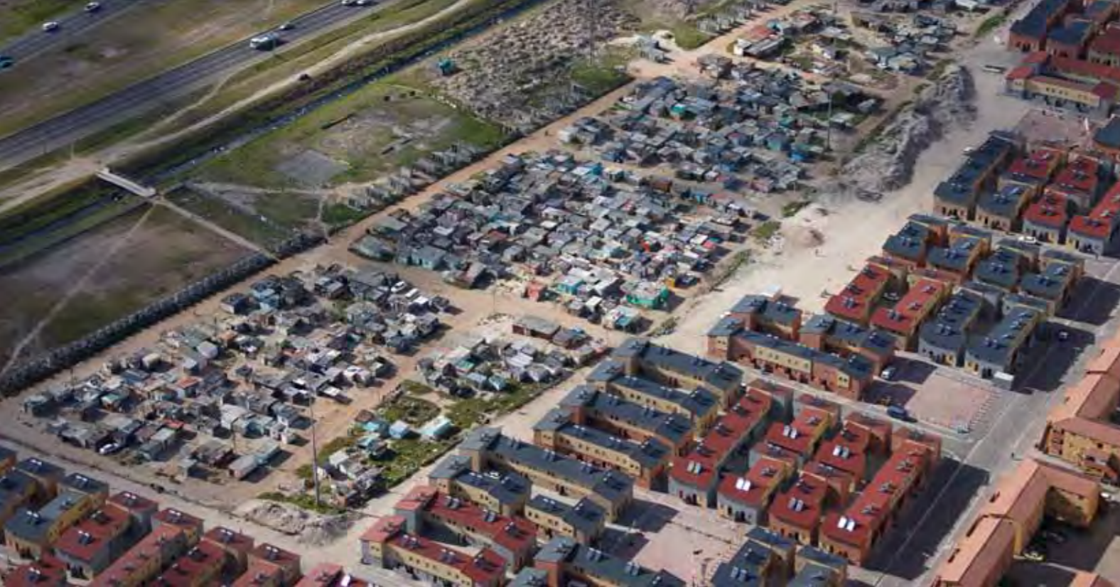
The N2 Gateway Joe Slovo Project demonstrates how the Department of Human Settlements is pushing for quality housing, rather than concentrated slum-type typologies. Photo supplied by HDA
