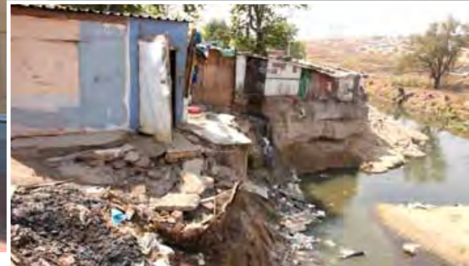
Homes built along the Jukskei River in Alexandra.
